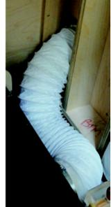
**NOTE:** Although all Mini One machines are ready to connect 4" (100 mm) exhaust hose and hose termination, they are not included in the standard shipment and must be ordered separately.
